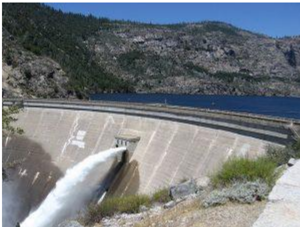
Hydroelectric power. (Photo: O'Shaughnessy Dam,
